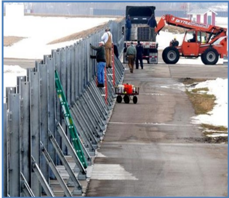
Figure 3-7: Installation of removable floodwall
